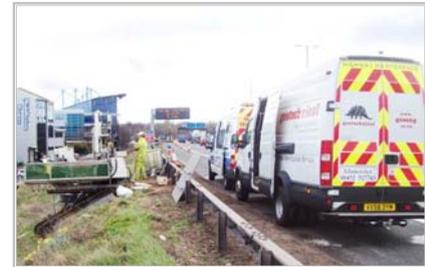
also install a range of instruments in the boreholes including inclinometers, extensometers, standpipes and piezometers. We have a dedicated monitoring team, who can read the instruments and feed the data back in a variety of formats, as required.
